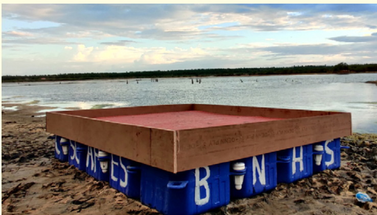
The platforms fixed on floats. The boards of the structure were made of waterproof wood; gaps were created to provide rainwater drainage
