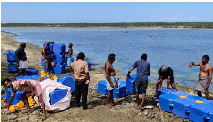
Assembling and setting up of the floating docks
