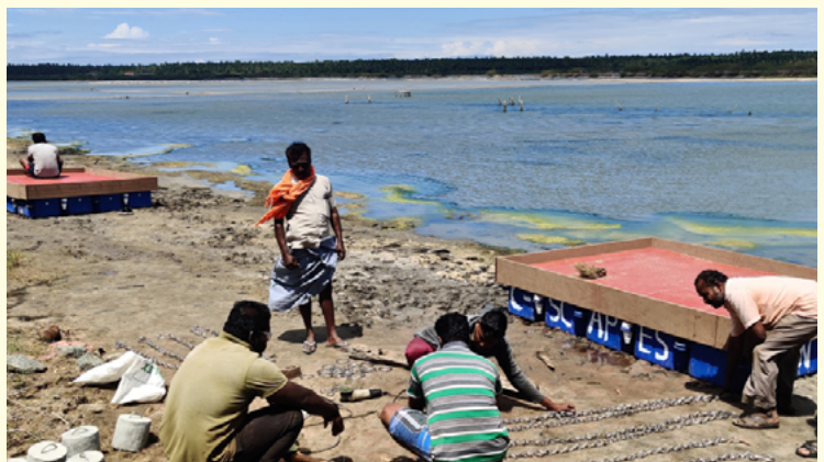
Concrete blocks weighing 3.5 kg were attached to metal chains (8 ft) fixed to the floats to provide anchorage
