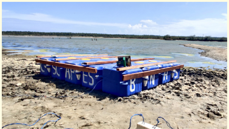
Wooden frame to be fixed on atop of the floats
